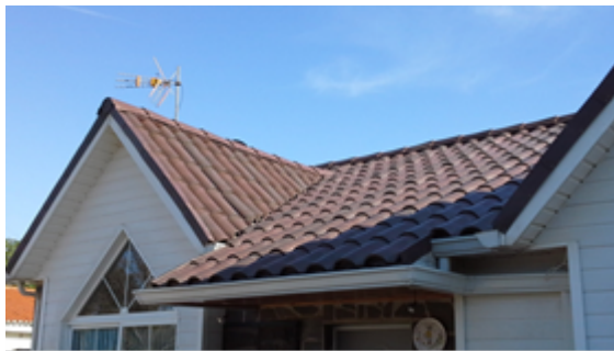
The Roofeco Spanish Rooftile in situ
